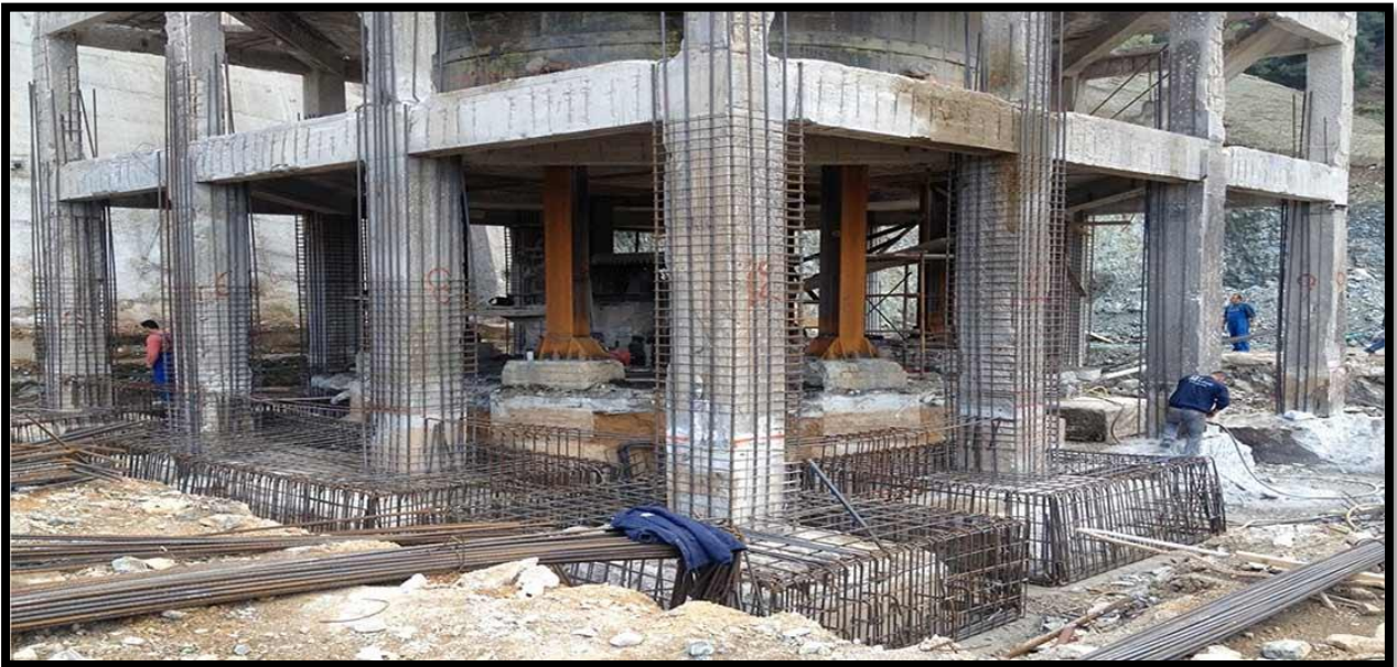
Fig.93 Seismic retrofitting of Buildings
