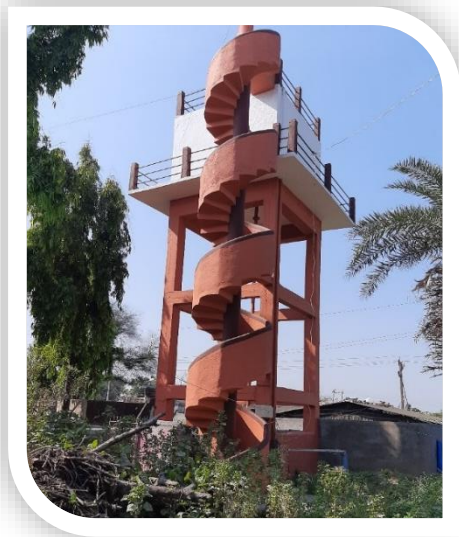
Fig.26 Overhead water Tanks 30,000 lit / 50,000 lit
