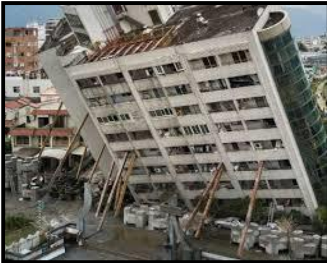
Fig.36 Soil liquefaction
