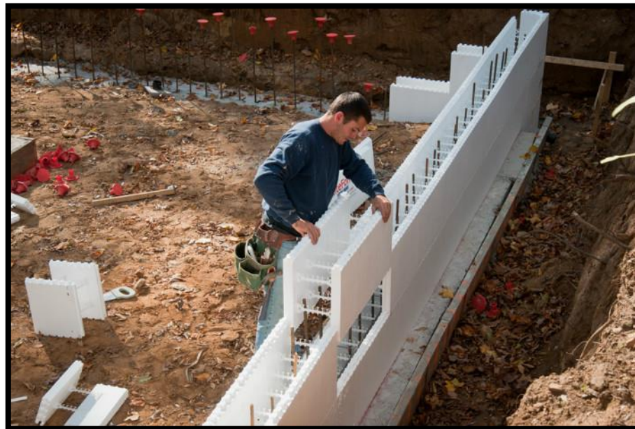
Fig.101 Insulating Concrete Formwork (ICF) Technique
