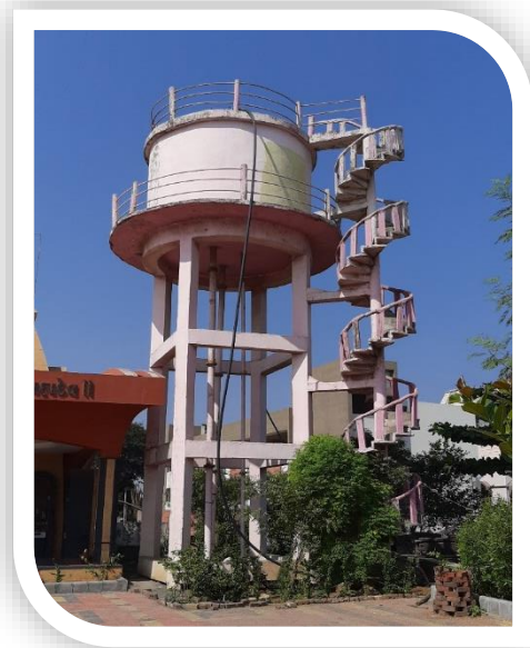
Fig.26 Overhead water Tanks 30,000 lit / 50,000 lit
